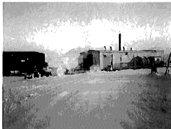
Eco Waste Solutions unit at CFB Alert located in building on base
