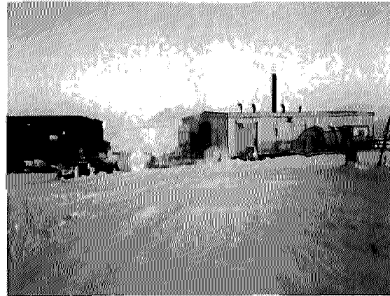
Eco Waste Solutions unit at CFB Alert located in building on base
